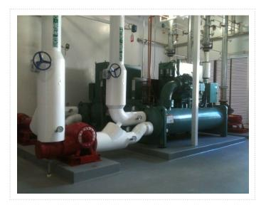
If possible, consider changing to a closed-loop system with a cooling tower, or otherwise, integrate the compressor cooling with another chilled water loop, like fermenting cooling. This chilled water loop is particularly effective when the brewery has several water cooled units. A small bleed will be needed for hygiene reasons.
