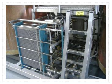
Make sure the heat exchangers are well maintained and regularly check the meter readings of the water flow. Pollution of the heat exchanger will negatively affect the heat transfer and cause an excess of water flow.
