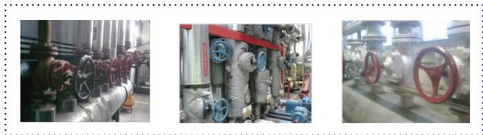
In many facilities, personnel will leave the flanges and valves uninsulated while insulating the pipe systems. Often the flanges are left bare, to avoid undetected leaks that may corrode the flange bolts. However, molded box insulation with inserts in the bottom of the box provides early warning of any leak. Non-insulated flanges and valves also introduce temperature stress, which may cause the leaks. Therefore, flanges and valves should never be left uninsulated.
